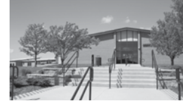
Elkhorn Campus 400 County Road H Elkhorn, WI 53121-2046 262.741.8200
