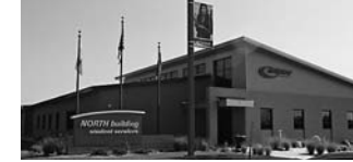
Elkhorn Campus 400 County Road H Elkhorn, WI 53121-2046
