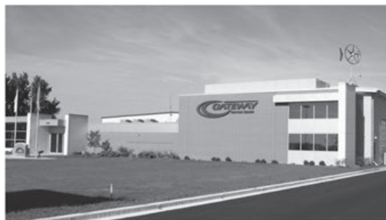
Horizon Center for Transportation Technology 4940 - 88th Avenue Kenosha, WI 53144
