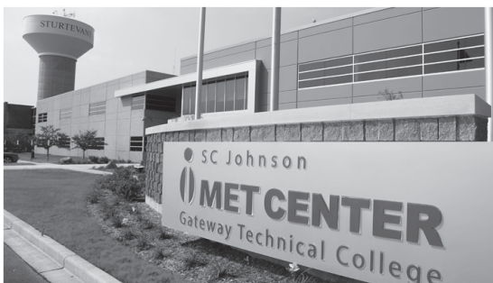
SC Johnson iMET Center 2320 Renaissance Blvd. Sturtevant, WI 53177
